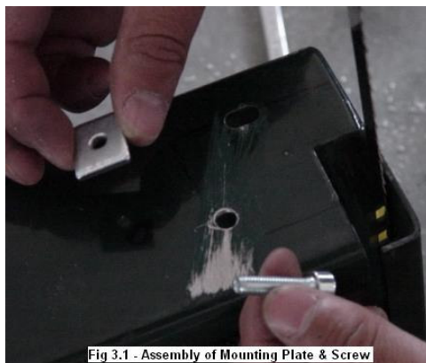
Fig 3.1 - Assembly of Mounting Plate & Screw
